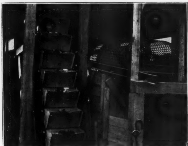
Scalping Screen and One of Elevators
